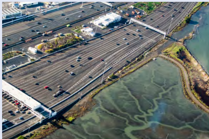
Essential Bay Area infrastructure, like the onramp to the Bay Bridge pictured here, lies close to the Bay shoreline and is vulnerable to sea level rise.
